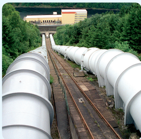
Water shoots down from a high reservoir through these conduits onto the blades of a turbine.
