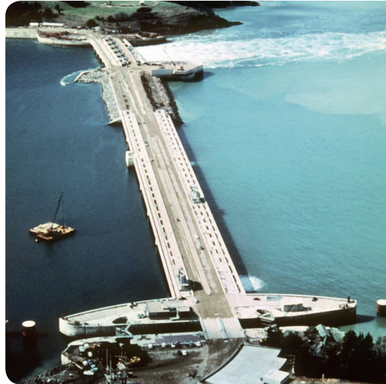
Tidal current drives the turbines at this tidal power plant near St. Malot, France. It was built in 1969. The Rance River serves as a storage pool.
