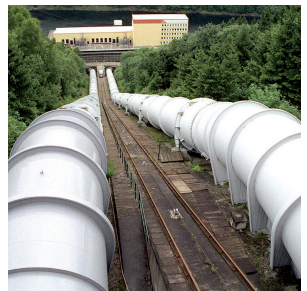
Hydropower plant with penstock pipes
